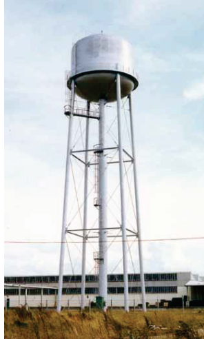
Figure C15.7-1 Multi-leg braced steel tank.
