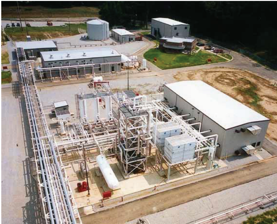
Figure C15.1-2 Steel pipe rack.
