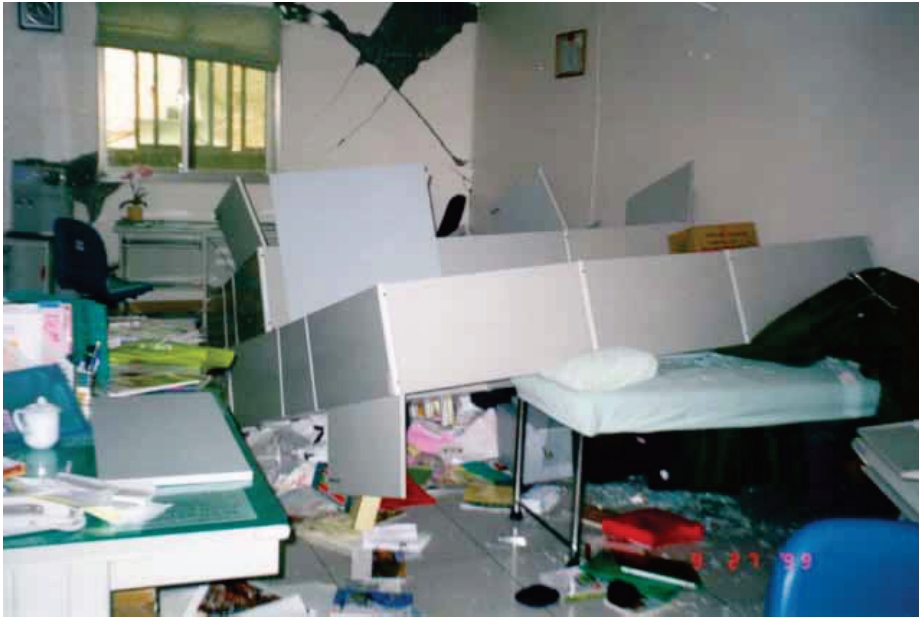
Figure C13.1-5 Toppled storage cabinets.
