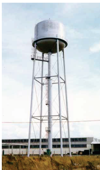
Figure C15.1-1 Steel multi-legged water tower.
