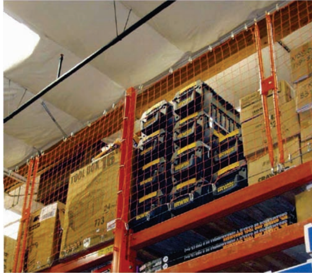
Figure C15.5-1 Merchandise restrained by netting.
